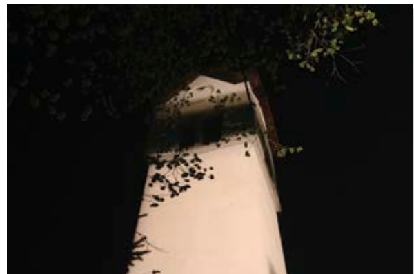
Shaded flight openings for bats in the belfry. Shading is enabled by the mask attached to a nature-friendly lamp and specially tailored to the façade of the building.
