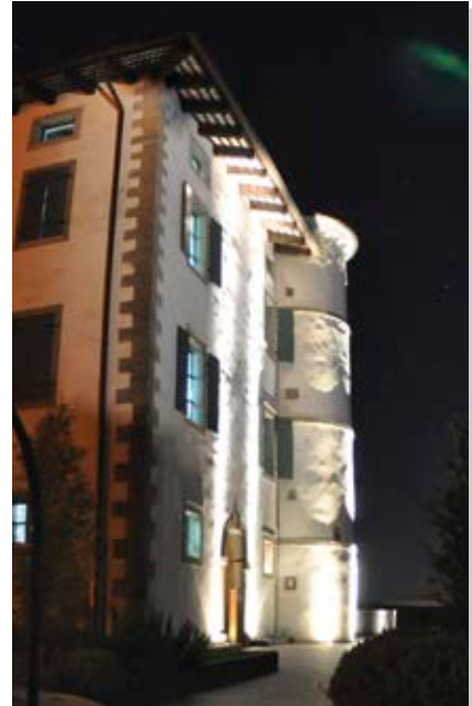
Lamps mounted right against the façade cause shadows which do not give the feeling of authenticity of the object.
