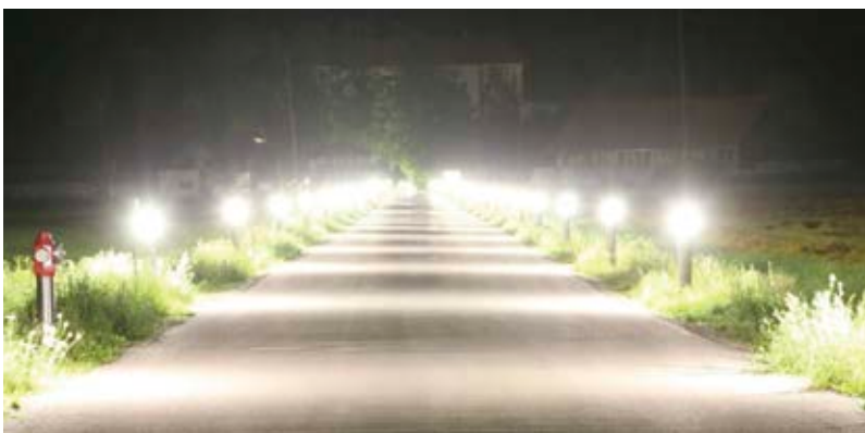
Access road to the cultural monument. This is an example of senseless and harmful investment: unbearable glare, light shining above the horizontal, and high maintenance costs. Also, the lawn around the luminaires will require manual mowing.
