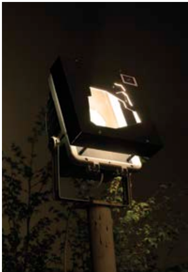
A shielded luminaire with an MH bulb with 3000 K and additional filter that blocks UV and blue light.
