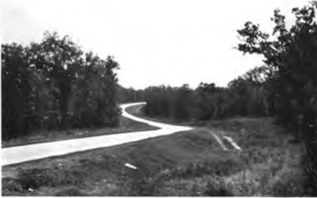
SHARP TURNED CURVES ON AN OLD-TYPE HIGHWAY
